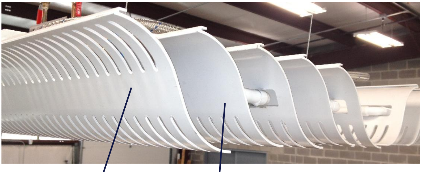
Standard Partial Slots, perimeter profiles are fully slotted and interior profiles are partly slotted
