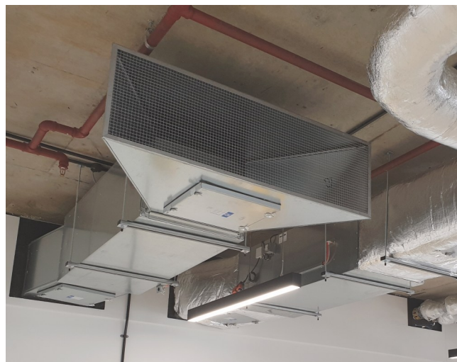
Typical application balanced supply and return air
